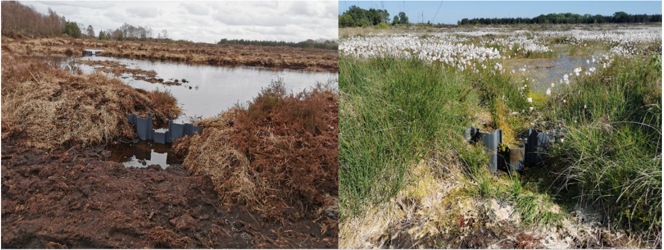
Figure 19: Cell bunding and plastic weir shortly after restoration (left, 2020) and after restoration (right, 2023)
