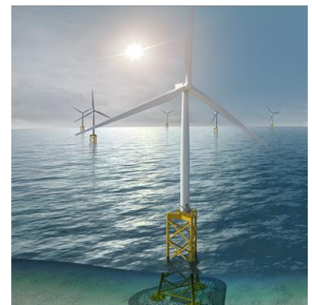
Figure 19 Fixed offshore wind turbine and foundation
