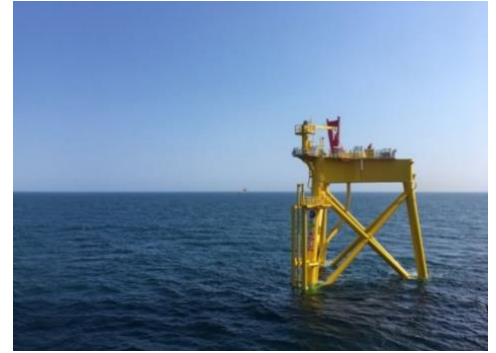
Figure 15 An Offshore platform
