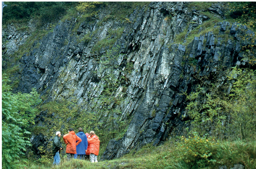
Fig. 5: Folded and fractured Mississippian limestone turbidite beds, Ape's Tor, North Staffordshire (photograph by J. Gluyas).
