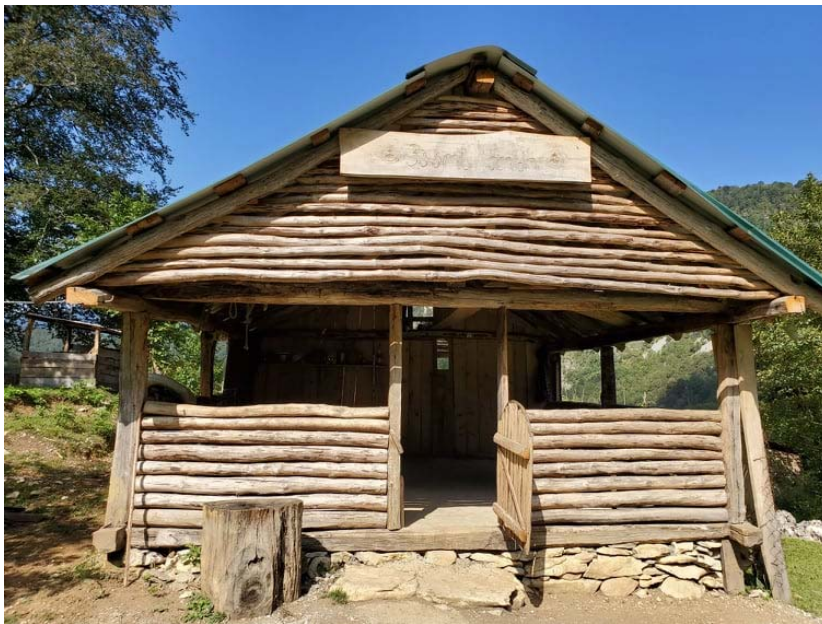
Picture 3: Vako Hut, located near the selected trail.
