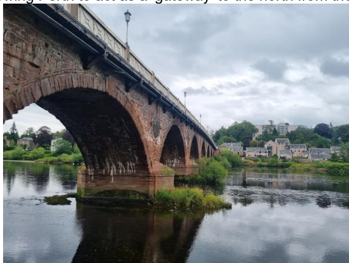
Figure 1: A85 Smeaton's Bridge
