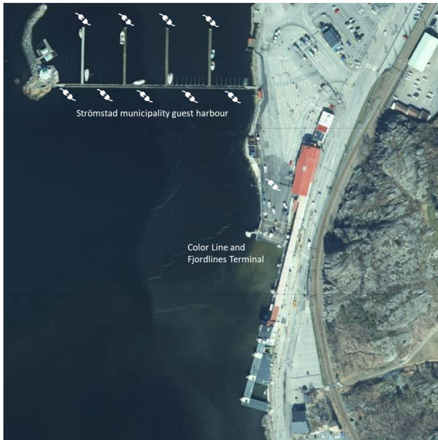
Figure 9. Torskholmen harbour area (aerial photo from Eniro.se)
