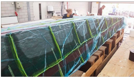
Fig. 14: Bridge beam during vacuum injection
