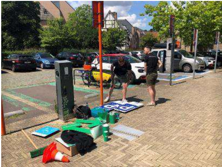
Figure 220 May 2022 – Installation of the alternative decoration of Ehub Park De Bruul
