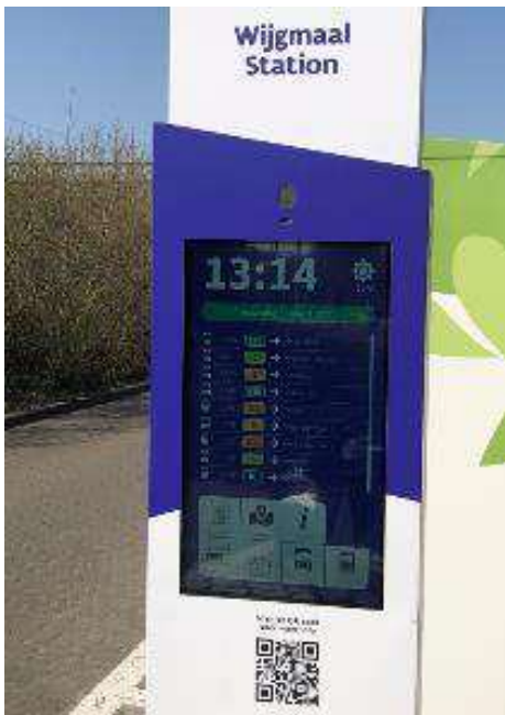
Figure 215 March 2022 – Connection of the digital pillar to the electricity network
