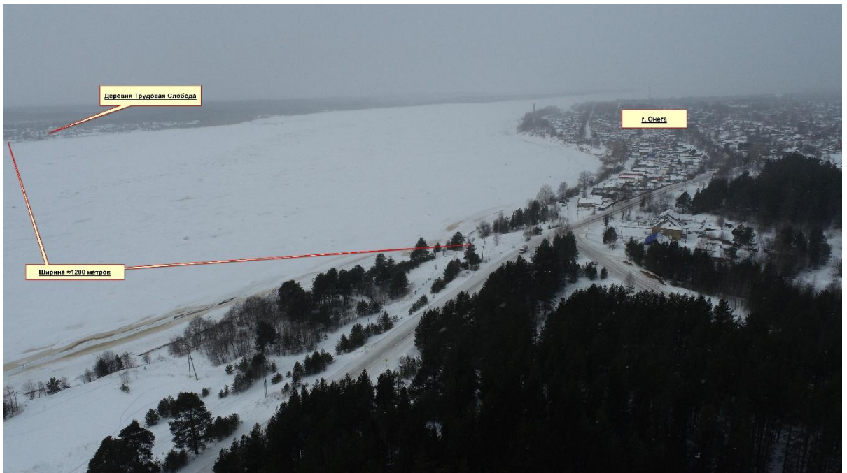
Picture. Location of the new bridge over Onega River between Trudovaya Sloboda and Onega town (Photo: Vyacheslav Lyapin, Domer PK)
