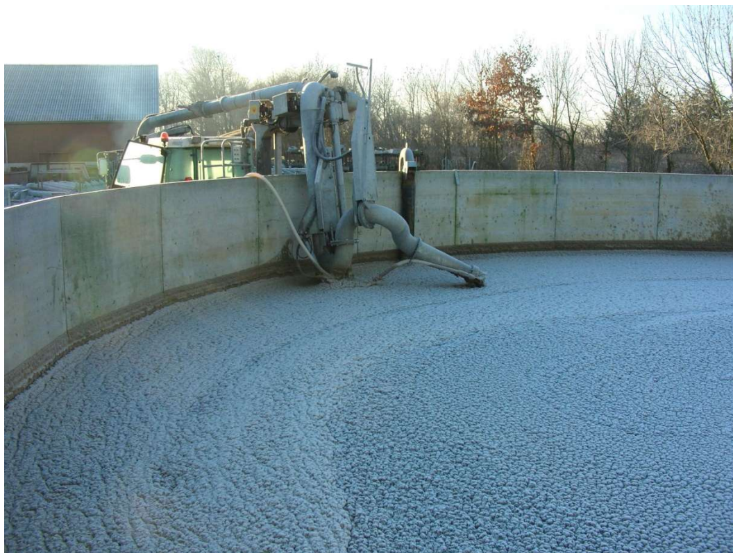
Acidification in the slurry storage is done in an agitation process, just before field application. Photo provided by HARSØ.
