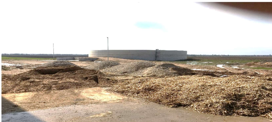
Newly build slurry tank at Dotnuva Experimental Farm, April 2016.
