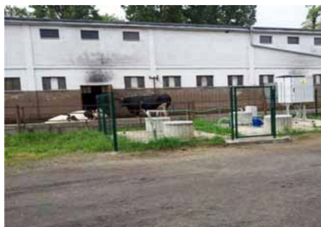
Figure 5. Experimental Farm in Falenty (ITP) in-storage slurry acidification automatic system before application on grasslands (in WP 4).
