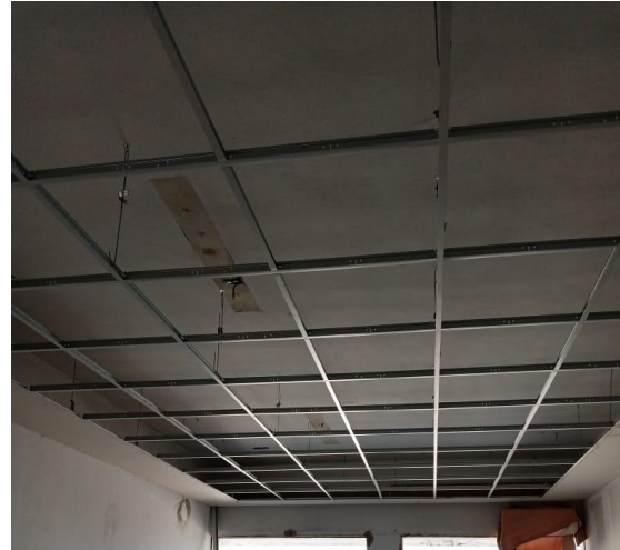
Figure 7: Ceiling thermal insulation installation
