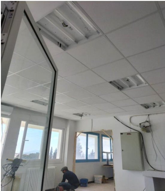
Figure 8: LED light installation
