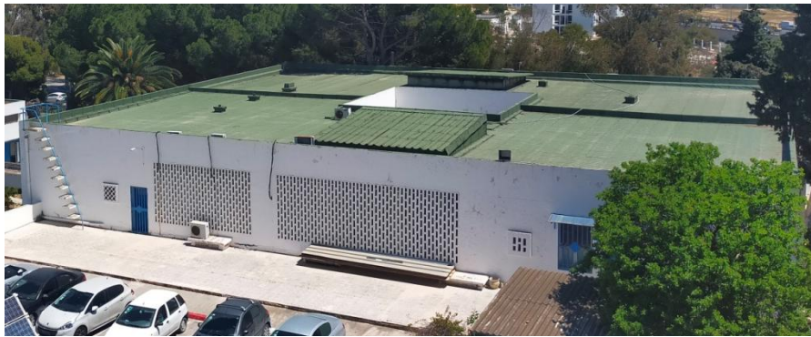
Figure 4: Thermal insulation at the roof of the administration building
