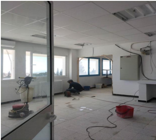
Figure 6: Double glazing installation
