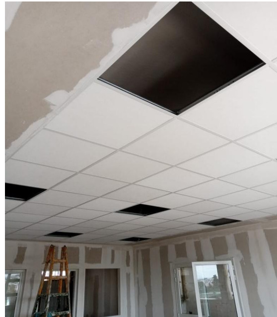
Figure 8: LED light installation
