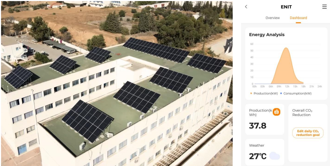
Figure 10: Rooftop PV power plant (Left); Monitoring system (Right)
