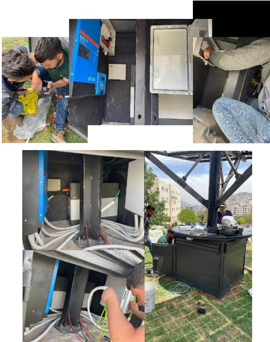
18-Then the DC/AC earthing was connected and lightning Pulsar
