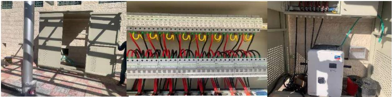
10-All the cables were installed in tranches and trunks for aesthetic image of the project and facilitate the maintenance work in future
