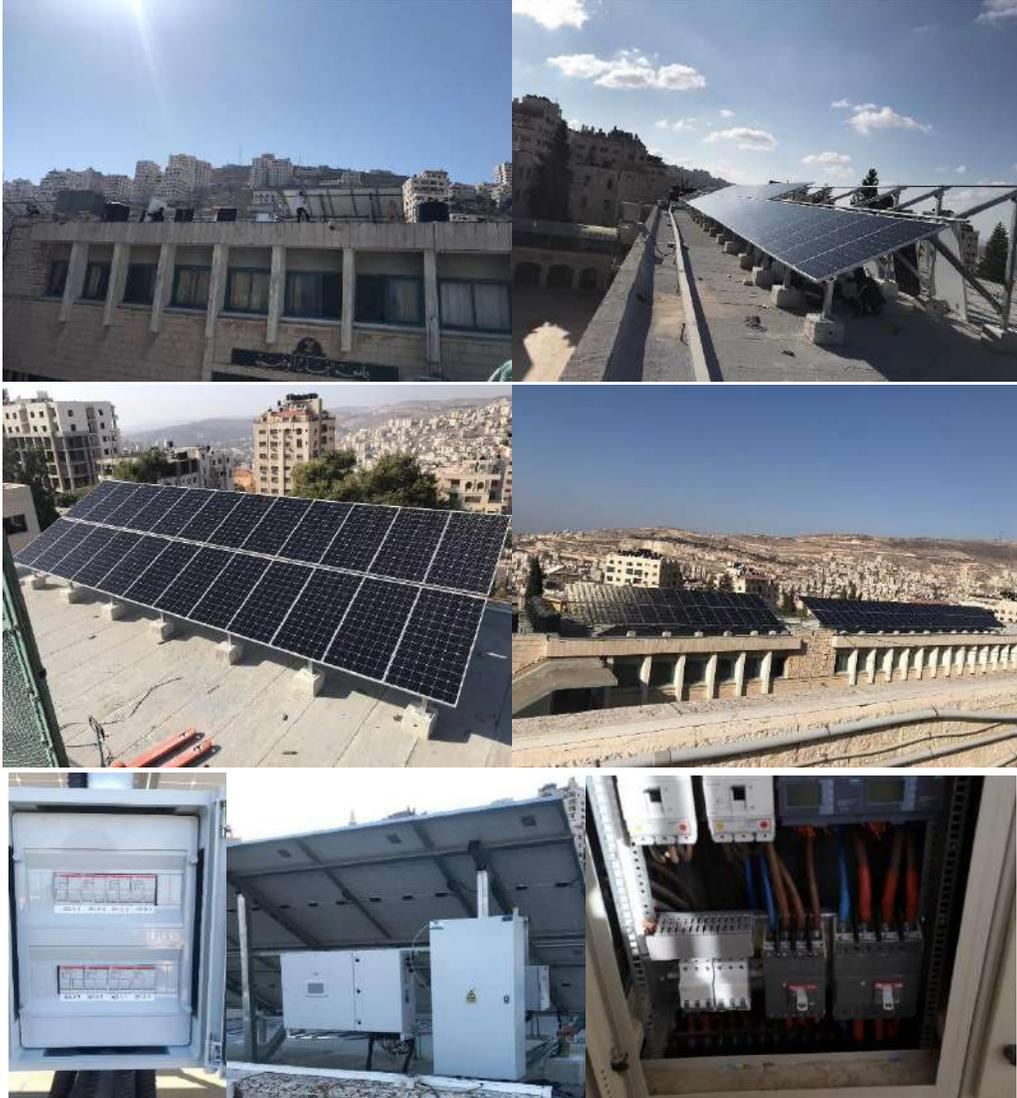
4- All the cables were installed in tranches and trunks for aesthetic image of the project and facilitate the maintenance work in future
