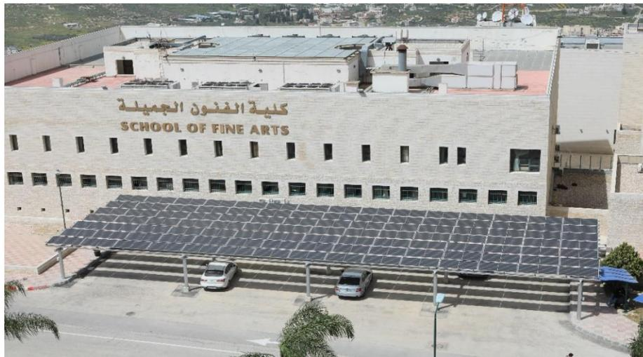
Fig.2 PV carport-new Campus PV system
