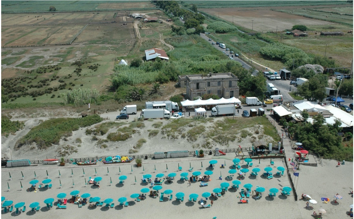
Figure 11. Access to the coastal area
