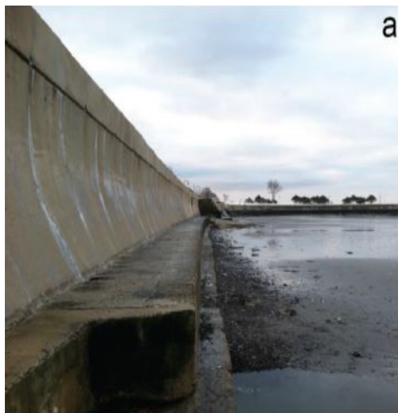
Figure 8. Seawall (Gittman et al. 2016)
