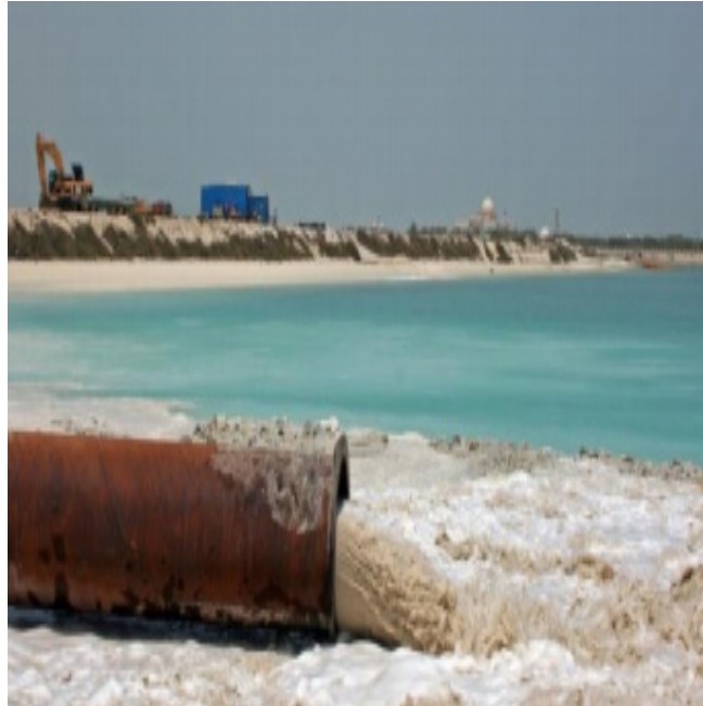
Figure 10. Sand bypass system (Loza, 2008)
