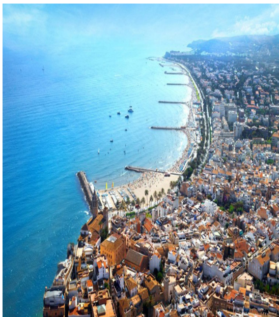
Figure 6. Transversal breakwaters (intersailclub.com).
