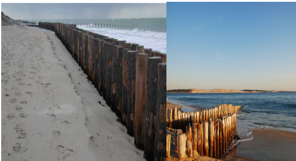
Figure 2. Stabilization of the lower beach by hydraulic piles
