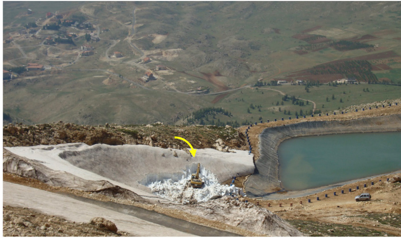
Figure 5. Excavating in snowpack results in loss of snow cover.
