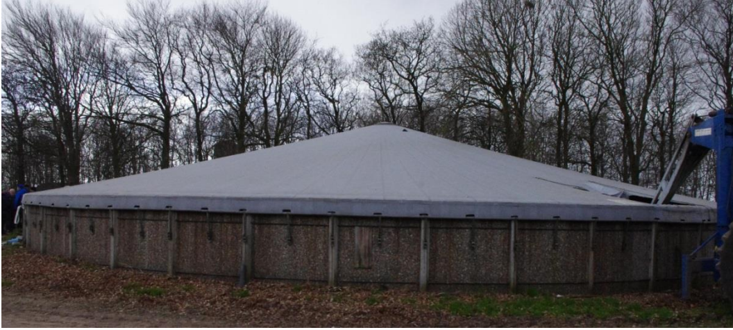
Figure 6. A slurry storage covered with tent. Denmark, April 2017. Picture by Kalvi Tamm.
