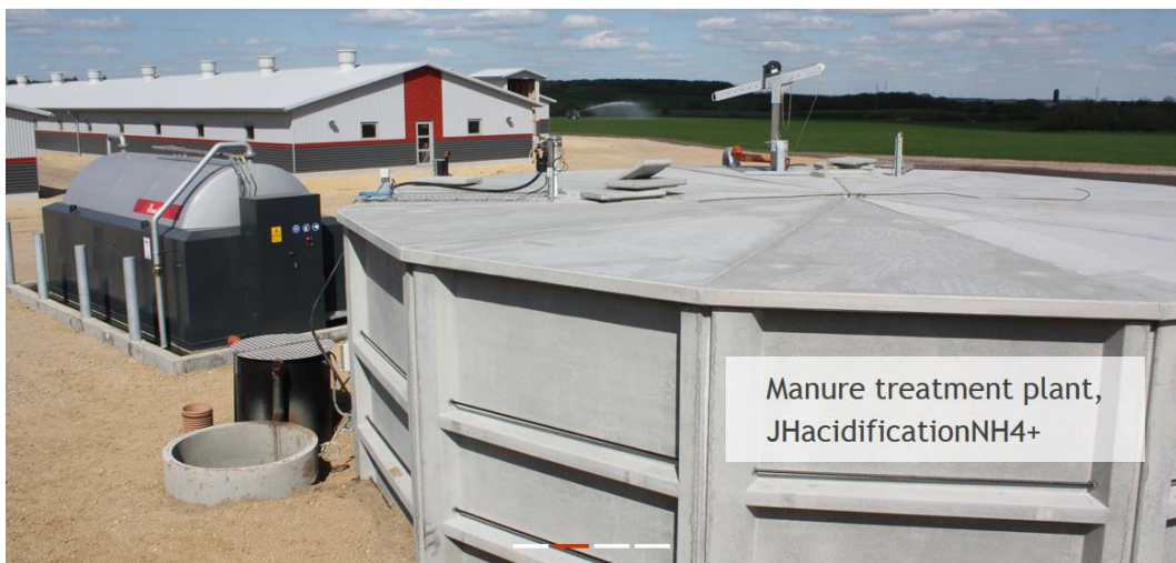
Figure 3. Acid tank (left) and processing tank near pig barn. (JH Agro)
