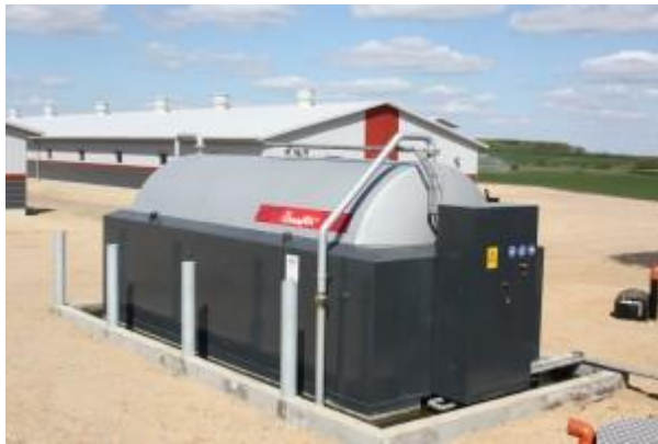
Figure 1. Sulphuric acid tank for in-house acidification (JH Agro)
