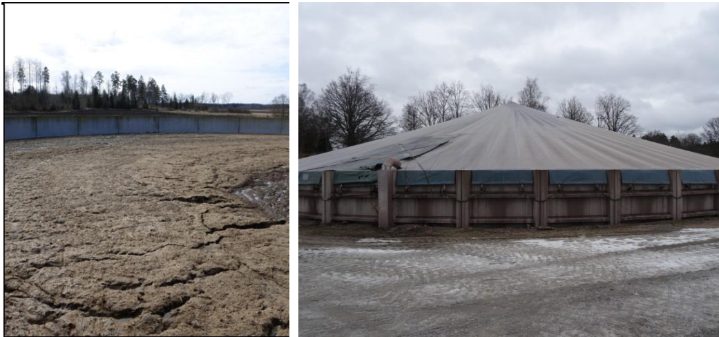
Figure 2-32. Slurry crust or roof as measure to reduce ammonia emissions on slurry storages. Filling is done below cover.
