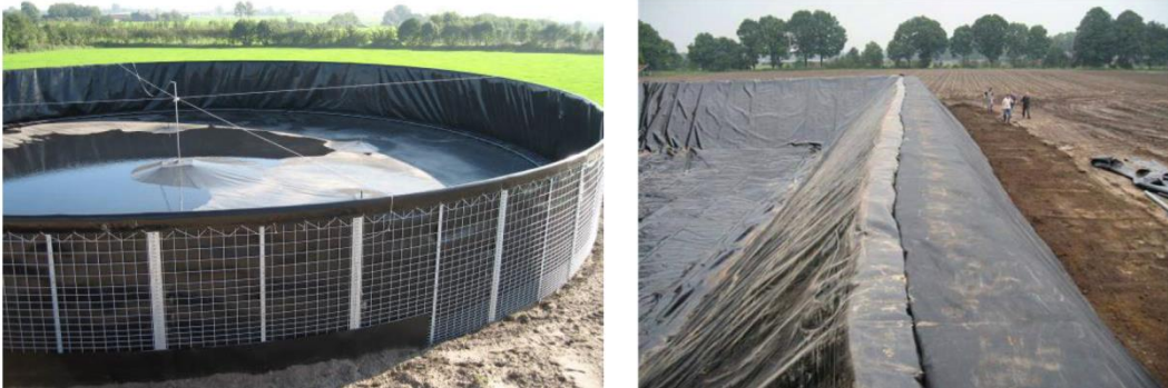
Figure 2-14. Slurry storage; container with roof (left) and open lagoon (right).
