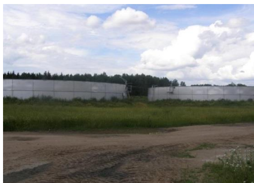
Figure 2-20. Slurry system in loose housing system for dairy cows (left) and concrete slurry storage tanks (right).
