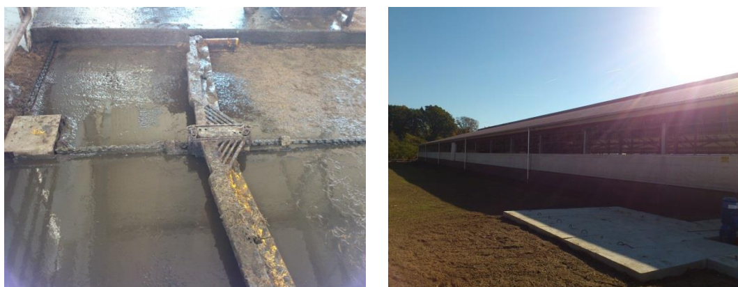
Figure 2-26. Slurry scraper on solid floor in walking alley (left) and modern free-stall cattle barn with intensive milk production (right). Photo: B. Lochowski, ITP.
