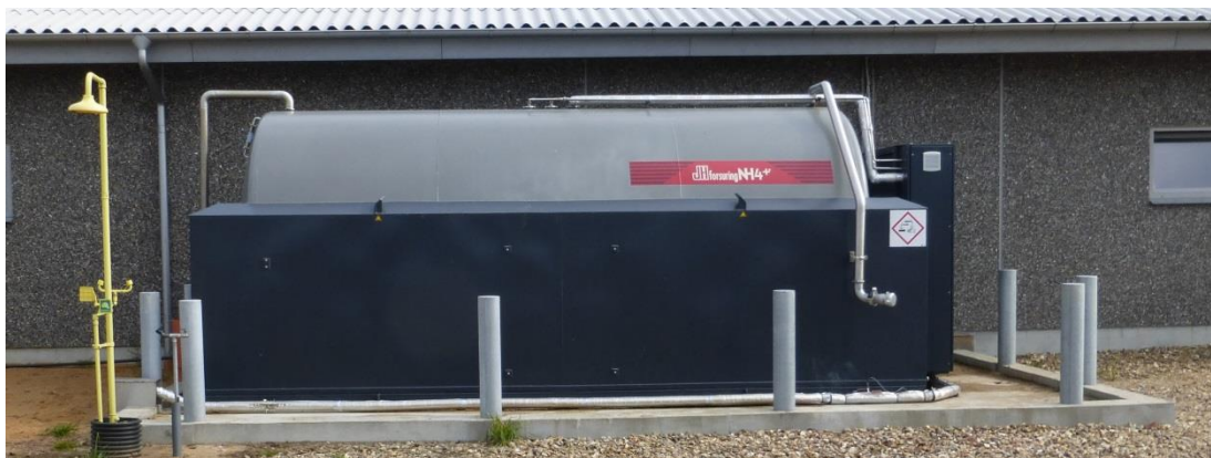
Fig. 5. Fixed acid tank surrounded by protective bollards, and with shower (JH Agro A/S).
