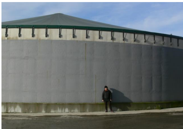
Fig. 13. Reinforced concrete tank with cover. Photo by: B. Łochowski
