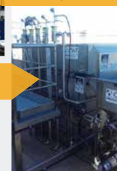
PROCAVI - Seville (turkey slaughterhouse)
