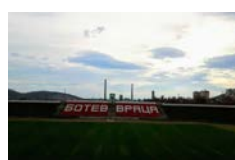
Stadionul "Hristo Botev" - Vratsa, Vratsa Stadium "Hristo Botev" - Vratsa, Vratsa Cod de identificare / Identification Code: 2774
