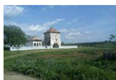
Fostul schit Deleni - Teslui, Deleni, Olt Former Hermitage Deleni - Teslui, Deleni, Olt Cod de identificare / Identification Code: 1718
