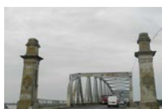
Podul de peste Olt - Slatina, Olt The Bridge over Olt - Slatina, Olt Cod de identificare / Identification Code: 1675
