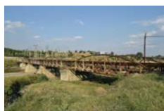
Podul metalic peste Râul Vedea - Alexandria, Teleorman Metal Bridge over the River Vedea - Alexandria, Teleorman Cod de identificare / Identification Code: 1514
