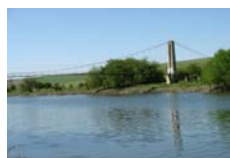
Podul de Frânghie - Belyanovo, Ruse Rope Bridge - Belyanovo, Ruse Cod de identificare / Identification Code: 2366
