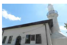
Geamia Mahmud - Hârșova, Constanța Mahmud Mosque - Hârșova, Constanța Cod de identificare / Identification Code: 1191
