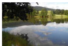
Barajul Gaganitsa - Berkovitsa, Montana Dam Gaganitsa - Berkovitsa, Montana Cod de identificare / Identification Code: 2189
