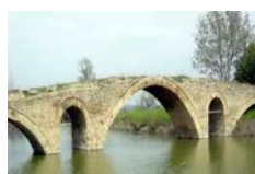
Vechiul Pod Roman de Piatră - Balgarene, Pleven The Old Roman Stone Bridge - Balgarene, Pleven Cod de identificare / Identification Code: 2232
