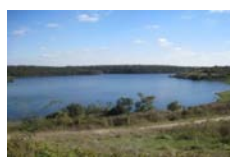
Barajul Antimovo - Tutrakan, Silistra Dam Antimovo - Tutrakan, Silistra Cod de identificare / Identification Code: 2438
