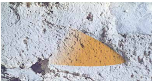
Builder's trowel and its imprint in the mortar of the wall of Lanišče fortlet
