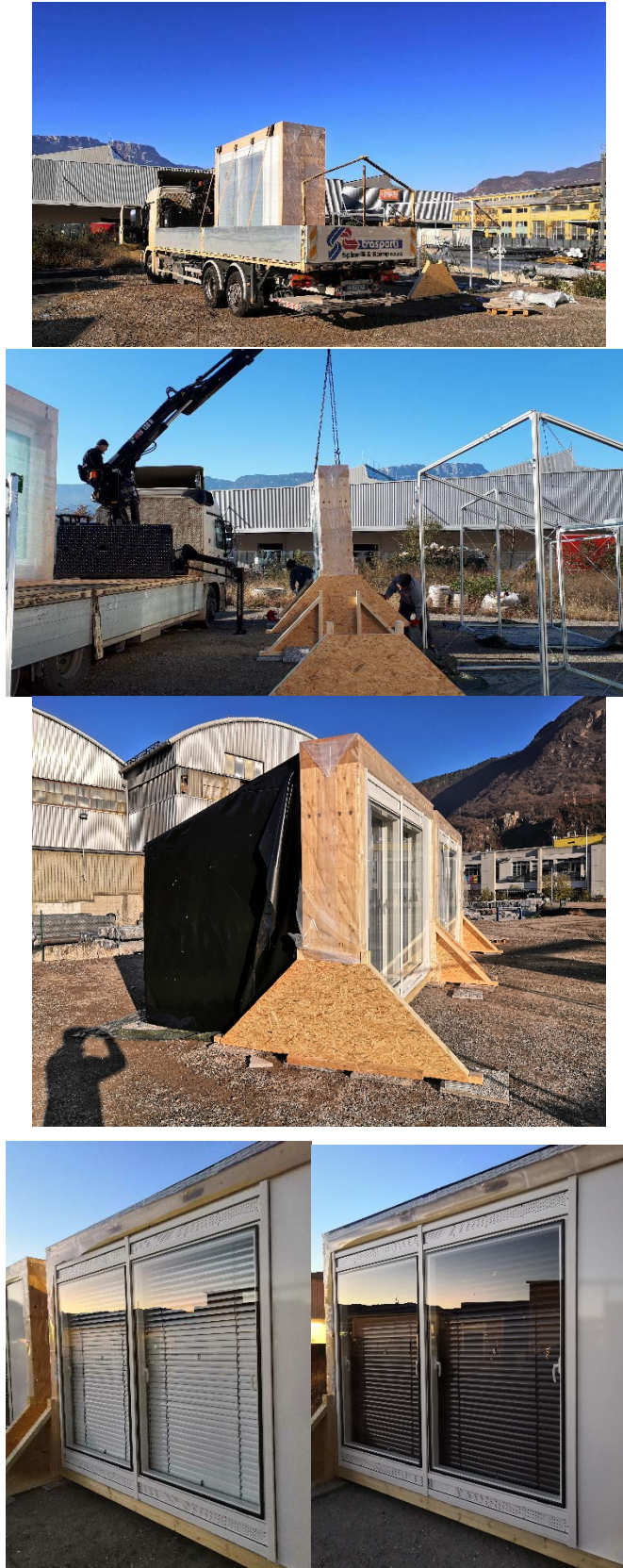
Figure 4: Transportation, installation of the FACEcamp façade specimen at EURAC outdoor lab.
