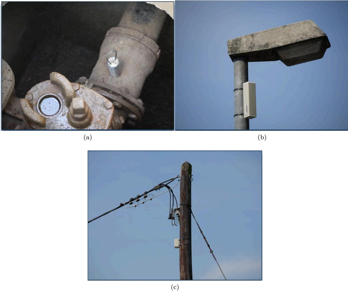
Figure 34: The ZoneScan monitoring system: (a) Loggers on a pipe, (b) Repeater set and (c) Alpha set
