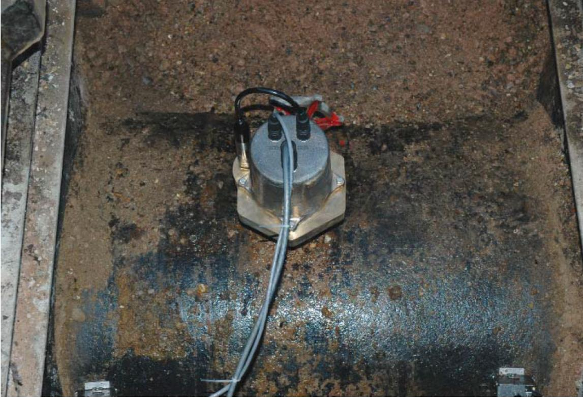
Figure 33: Trunkminder: Installation of head unit on trunk main.
